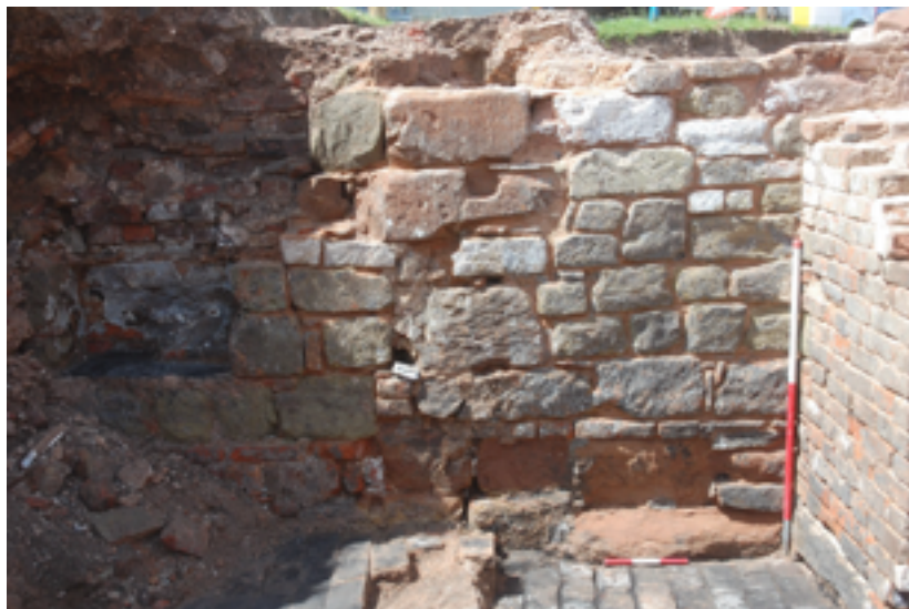
Figure 34: Sandstone wall No. 3 College Street CG24, facing west
