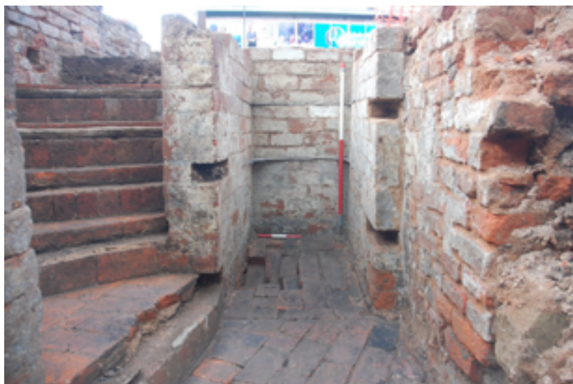
Figure 35: Staircase and pantry CG25 in No. 3 College Street, facing north
