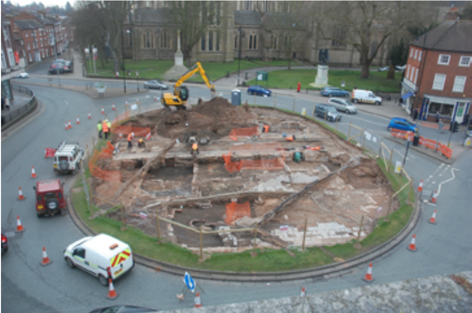
Figure 4: Machine excavation with traffic management in place, facing south
