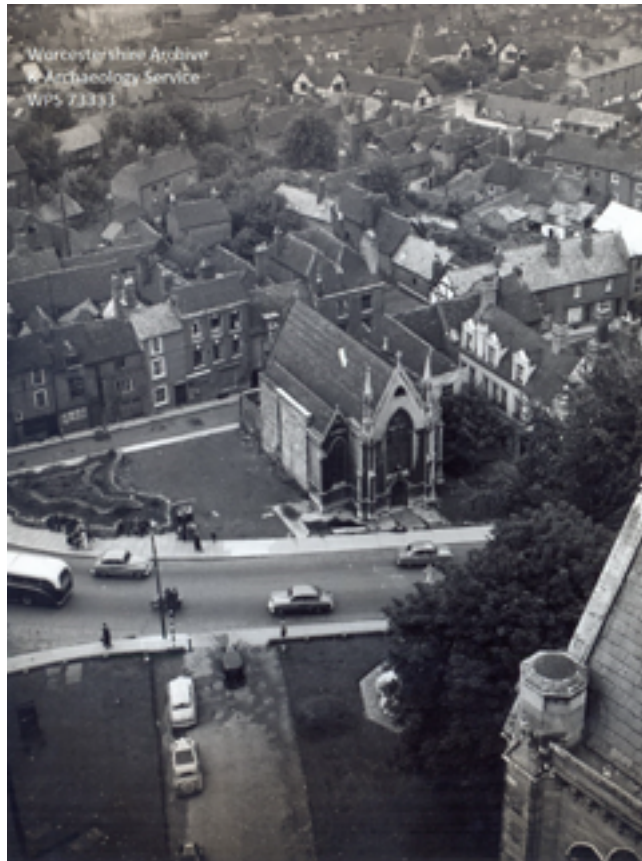
Figure 11: Buildings removed from west end of Lich Street (WAAS)
