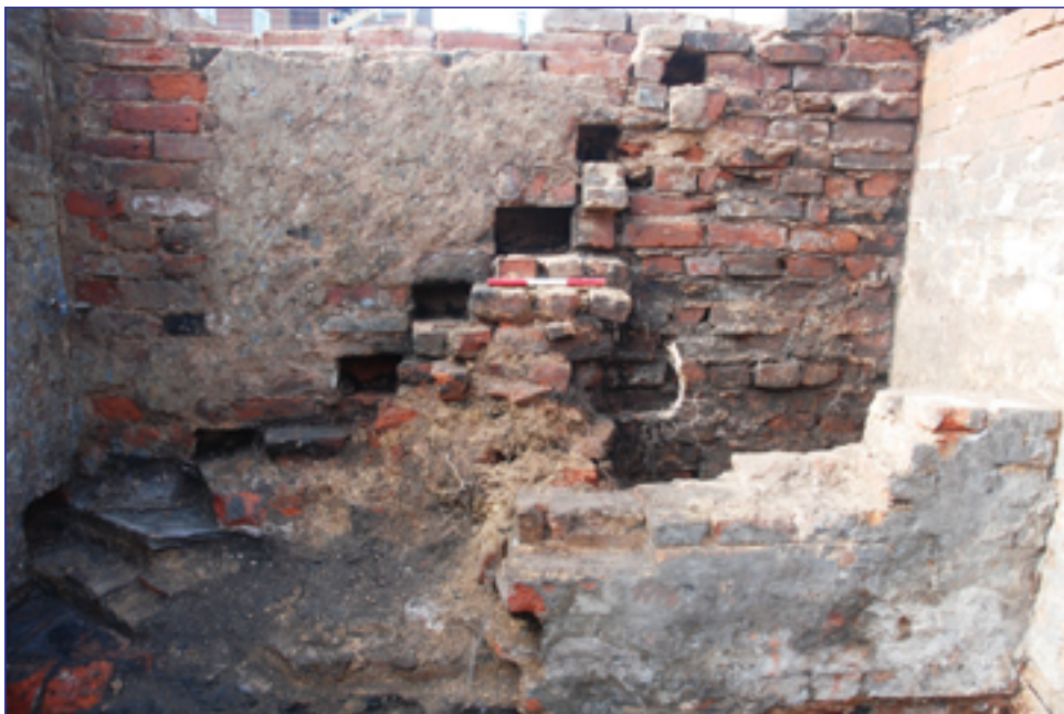
Figure 18: Staircase in No. 3 cellar (ecclesiastical stonework was in space behind wall in foreground)
