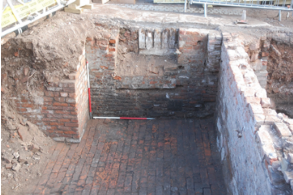
Figure 29: Cellar walls No. 4 Lich Street, facing north
